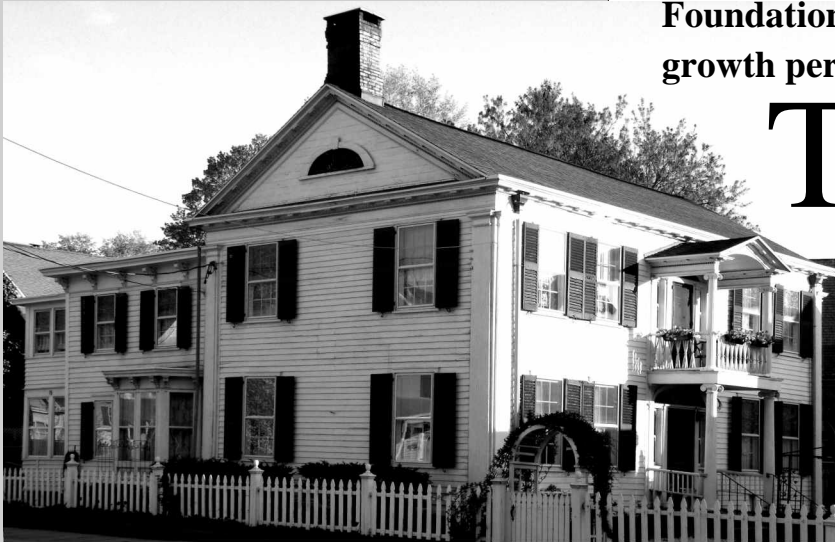
The Jeremiah Russell house with street corner Greek revival pedimented gable facing Ulster Avenue and Federal eave side entry facing Market Street has Italianate additions, all showing the influences of the entire growth period of Saugerties
