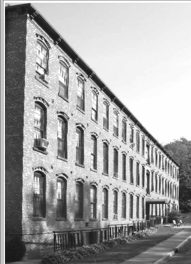
The west wall of "The Mill" with three floors of 21 arches each in their original 1887 condition
