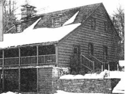
Early 20th century photo and current restoration of once common 18th century timber-over-stone bank house
