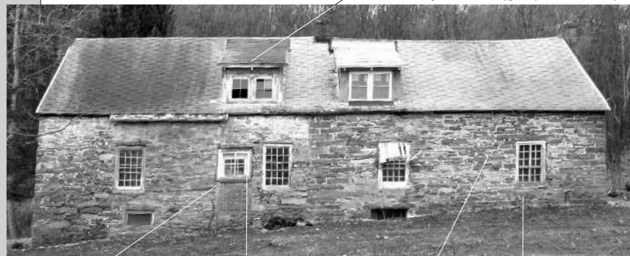
Mating seam of original house (random stone courses) Merging section (interim pre-center hall entry) Later expansion house (more formal stone shaping) 12 over 8 windows (late 18th century)
