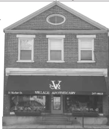
Rare Greek Revival store with Dutch cross course brick laid on bluestone water table band
