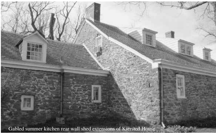
Gabled summer kitchen rear wall shed extensions of Kiersted House
