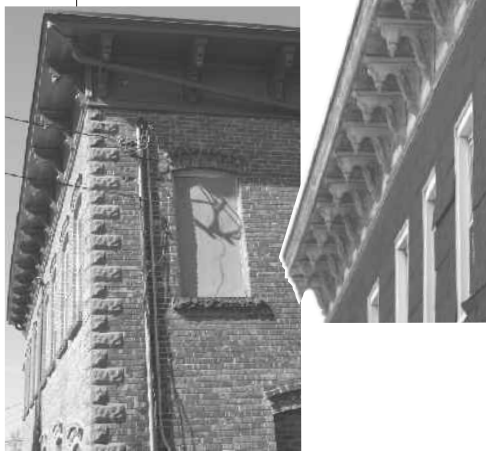
The bracketed cornice with broad frieze boards following the rake of the gable is a typical feature of the post Civil War Italianate style of Saugerties
