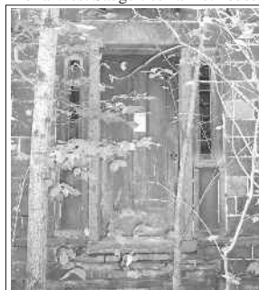
Unique stone framing on side lights of Jeremiah Russell Turnpike house
